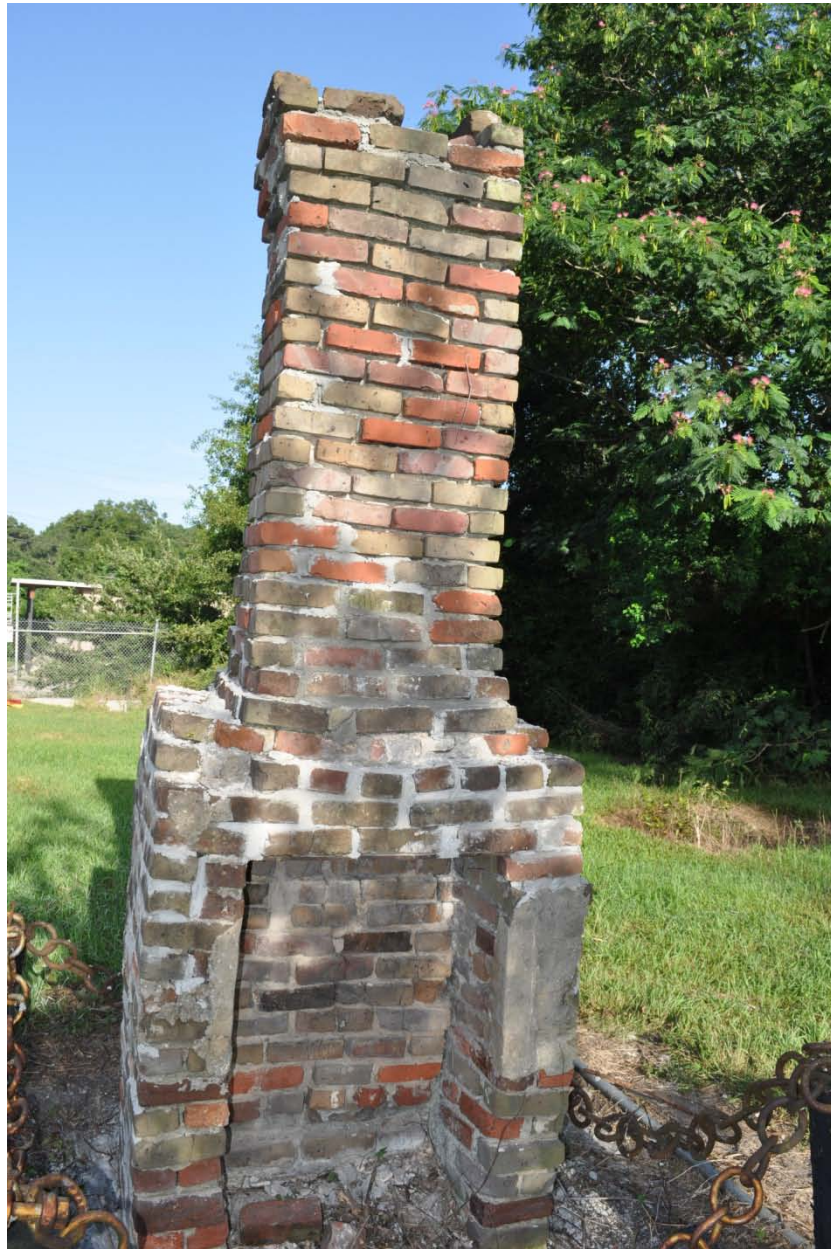
Figure 12 Peter Lee House Test Chimney After Repointing
