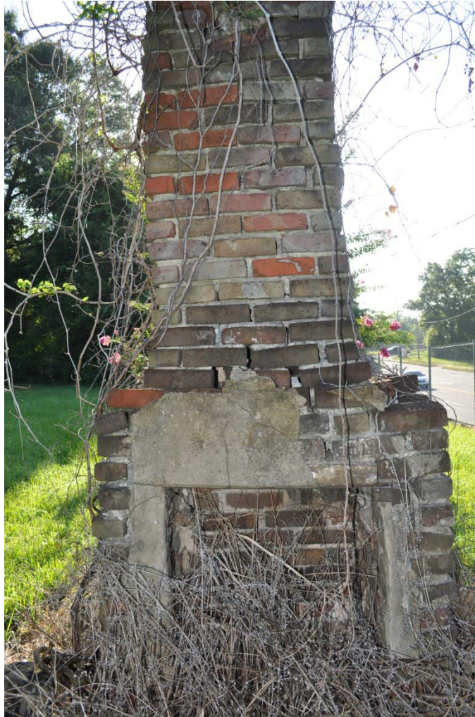
Figure 11 Peter Lee House Test Chimney Before Repointing
